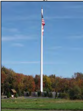
Stealth Monopole As Flagpole
