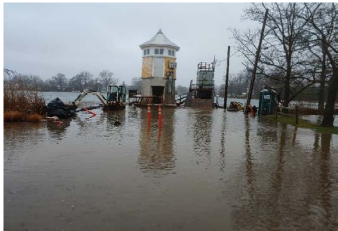
Figure 15. Meadow Pump Station flooded during a high tide on December 30, 2019. Photo Courtesy of Greenwich.
